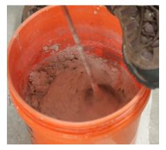
**Mix the mortar** specified for your tile according to the directions on the bag. Mortar is caustic, so be sure to wear protection. Mortar can't be used once it dries out, so don't mix too much at once.
