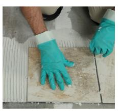
Once you've confirmed you have the right consistency in your mortar, **align** the first tile with your chalk lines and press firmly into the mortar. Place two spacers along the side at either end and set your second tile by aligning the edge, hinging it down and slightly twisting it back and forth.
