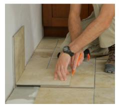
Now you're ready to cut tiles to fill the space along the wall. Place two tiles up against the wall to allow for expansion and grout (at least 1/4"). Then place the tile to be cut directly over the last set tile. Finally, place a marker tile on top of the tile to be cut so that it touches the upright tiles. Trace the edge of the marker tile to mark the tile below.
