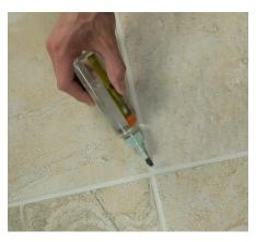
After 72 hours, apply grout sealer along grout lines, making sure to wipe up any excess within ten minutes.
