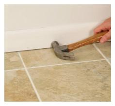
Finally, **cover the expansion gap** along the walls with moulding or matching bullnose tile and install any desired thresholds between neighbouring floors.
